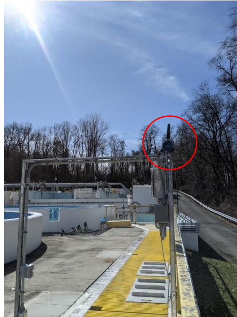
Installation by Sedimentation Tanks
