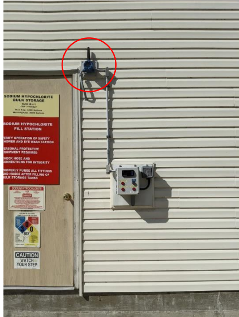
Installation at Storage Sheds
