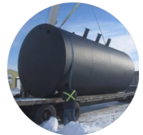
ROUND HORIZONTAL TANK MONITORING
