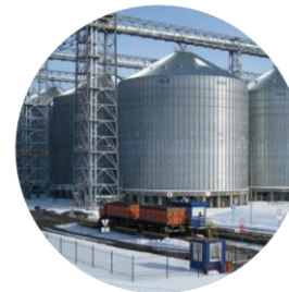
SILO HEIGHT DISPLAYS
