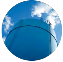
Tank Height Measurement
