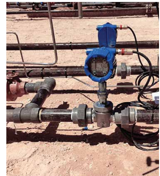
Photo courtesy of Turbines, Inc. PD6830 Mounted on Turbines, Inc. Flow Meter
