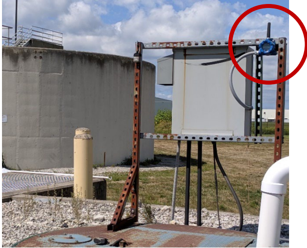
PDW30 Field Unit Transmitting Two Measurement Signals
