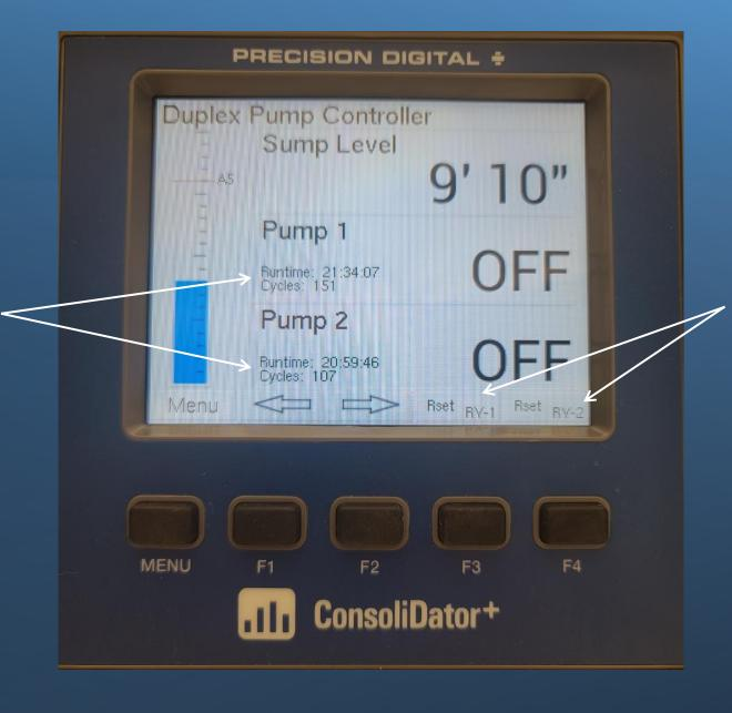
These "Soft Keys" are there to allow an operator to reset the "Runtime" and "Cycles" of "Pump 1" or "Pump 2"
