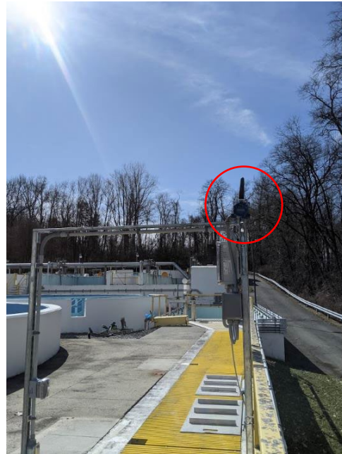
PDW90 Field Unit Installation at Open Channel Flow
