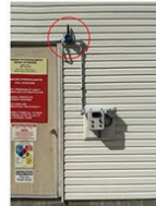
PDW90 Field Unit Installation at Storage Building
