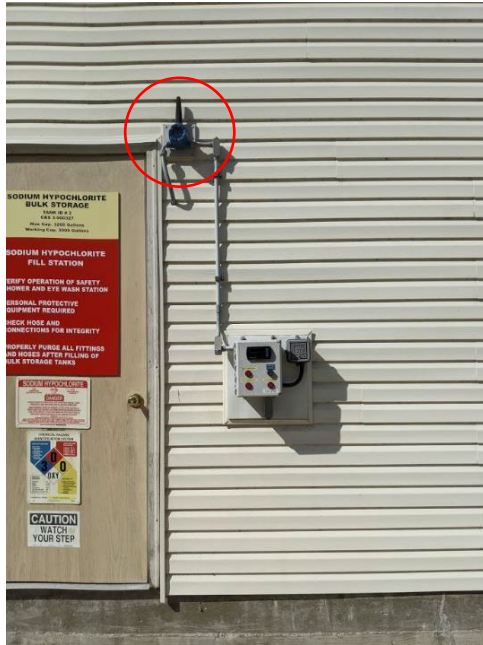
PDW90 Field Unit Installation at Storage Building
