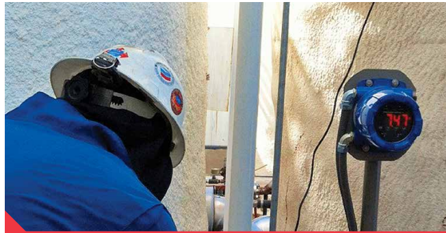
Modern equipment features such as through-window buttons allow operators to configure instruments without removing the cover in hazardous areas.
