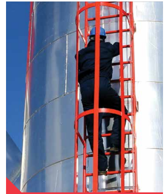
A remote display eliminates the need for operators to climb tanks for level readings.
